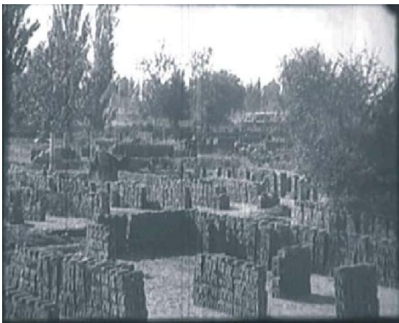
Fig. 2: Drying bricks in the middle of the city. (Kyzylorda, 1925) Source: TsGAKFDZ RK
